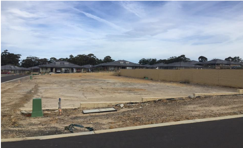
Island Point, NSW – 25 units to be constructed
