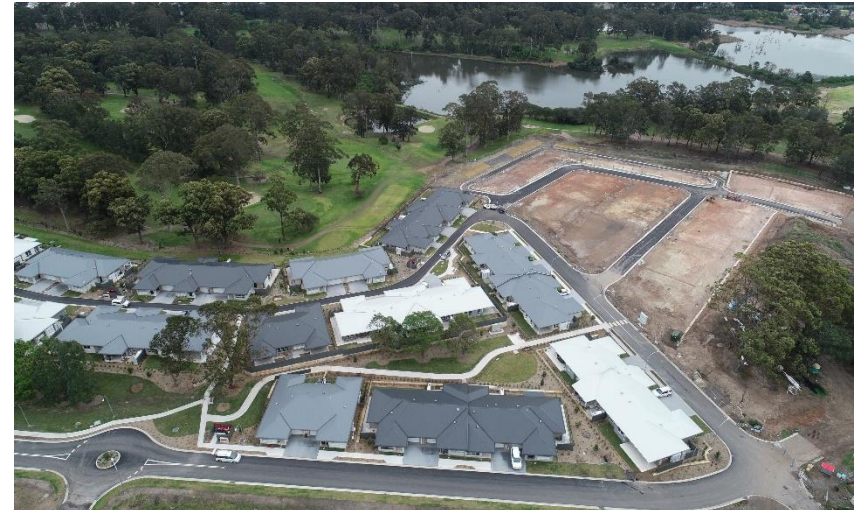
Newcastle, NSW – 37 units to be constructed
