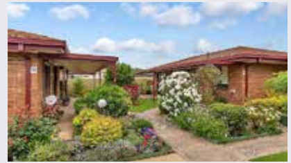
Aveo Crestview 136 Fosters Road, Hillcrest
