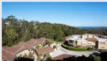
Aveo Minkara Resort 10 Minkara Road, Bayview
