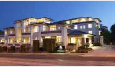
Sackville Grange 378 Cotham Road, Kew
